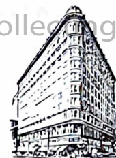
For two years, 20 Vacuettes have been used every night in the Phenian Building, San Francisco.
