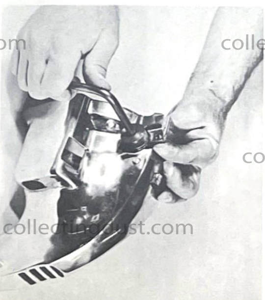
Figure 1-59. Using handle spring tool (SP123)
