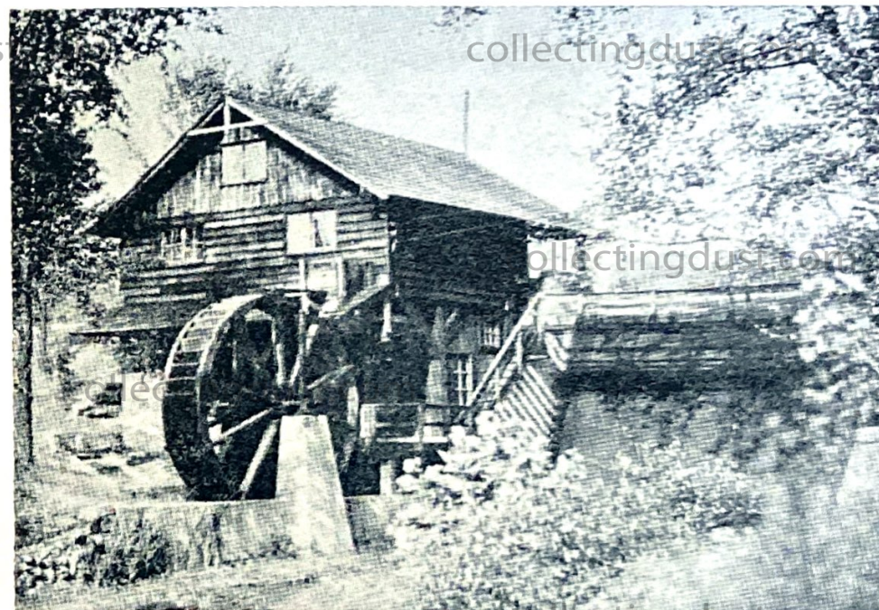
The first ball bearing mill wheel. The slightest trickle of water operates it.
